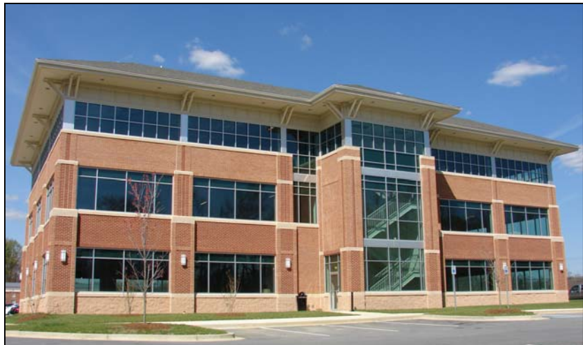
Fairview Center Building 2 Rear View
