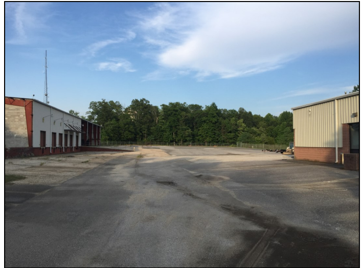
Warehouse and storage yard
